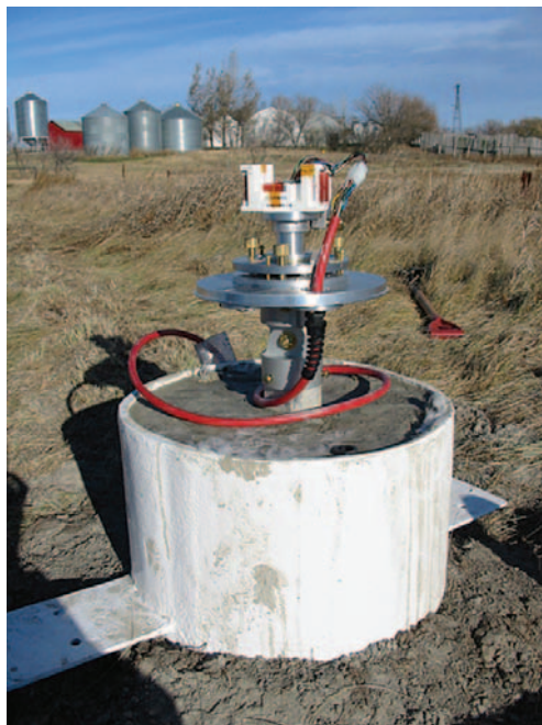
Fig. 13. Typical fluxgate magnetometer sensor head mounted in the concrete base of its protective silo (site: GULL).
