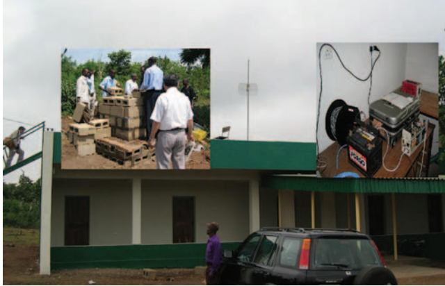
Fig. 8. Installation of the MAGDAS Instrument at Ilorin, Nigeria.
